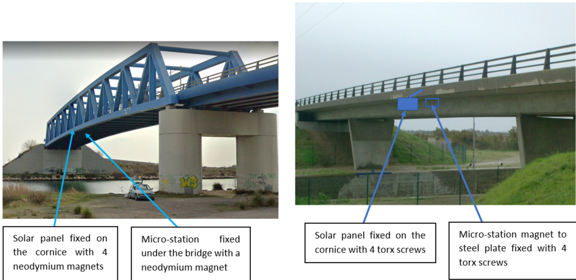
Figure 2: Description of the installation in the Rhône delta sites with Fos-sur-Mer on the left and Port saint Louis du Rhône on the right
